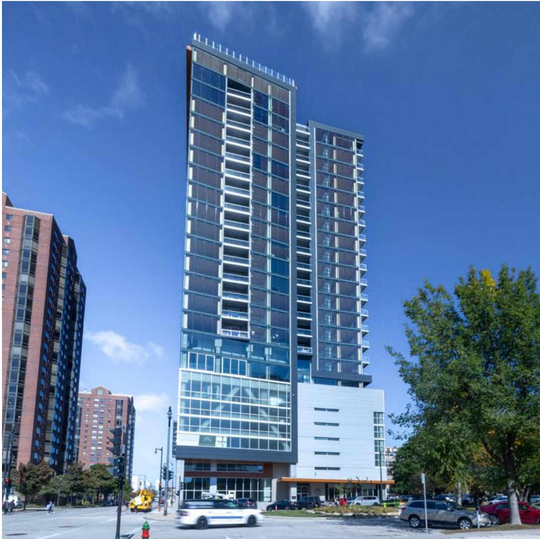
Figure 9: Ascent MKE in Milwaukee effectively uses materials where they are best suited. Here the first 6 storeys – with house the foyer, pool, and other amenities - are constructed from traditional reinforced concrete, with a 19-storey timber tower rising above.
