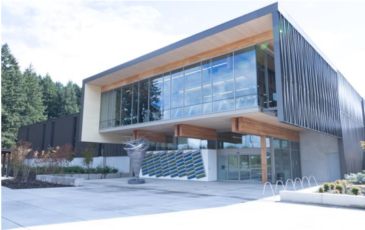
Figure 13: The Hidden Creek Leisure Centre in Hillsboro (Oregon) utilises an access floor and isolation mounts to minimise the transfer of vibration from the first floor gym.
