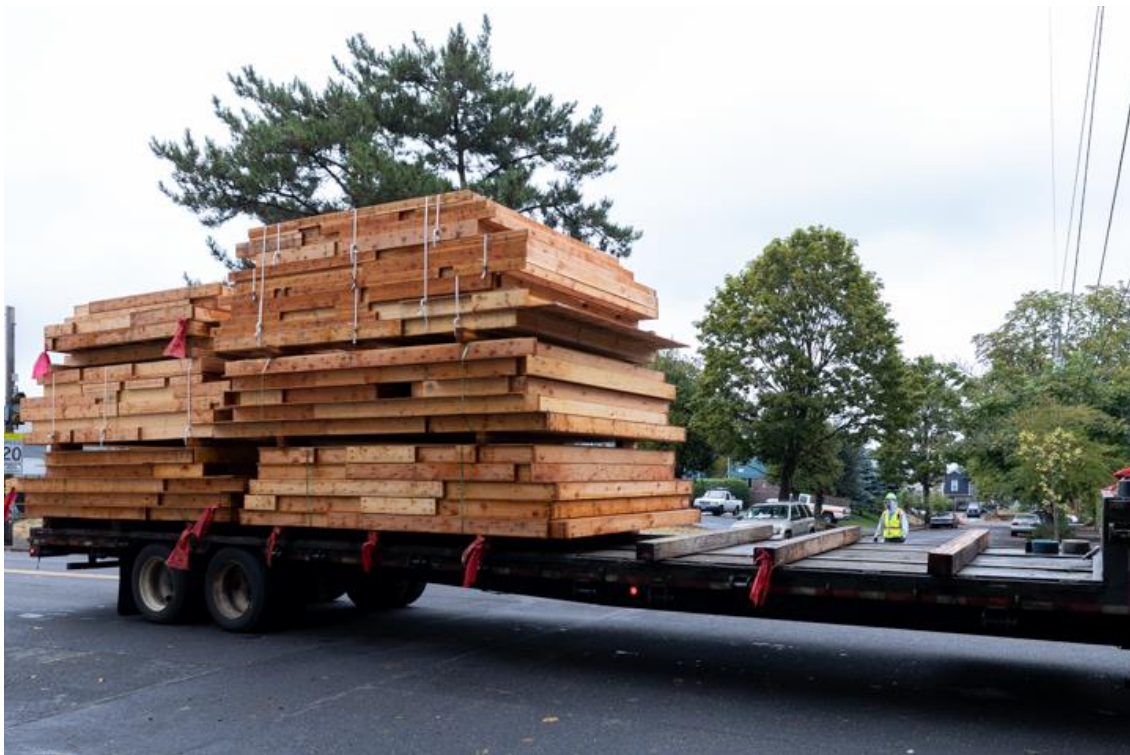
Figure 14: Prefabricated lightweight construction is a quickly growing form of timber construction in the USA. Unlike ‘stick built’ construction, this approach sees wall frames and floor cassettes prefabricated off site and delivered to site on the back of a truck as seen here in Portland, Oregon.
